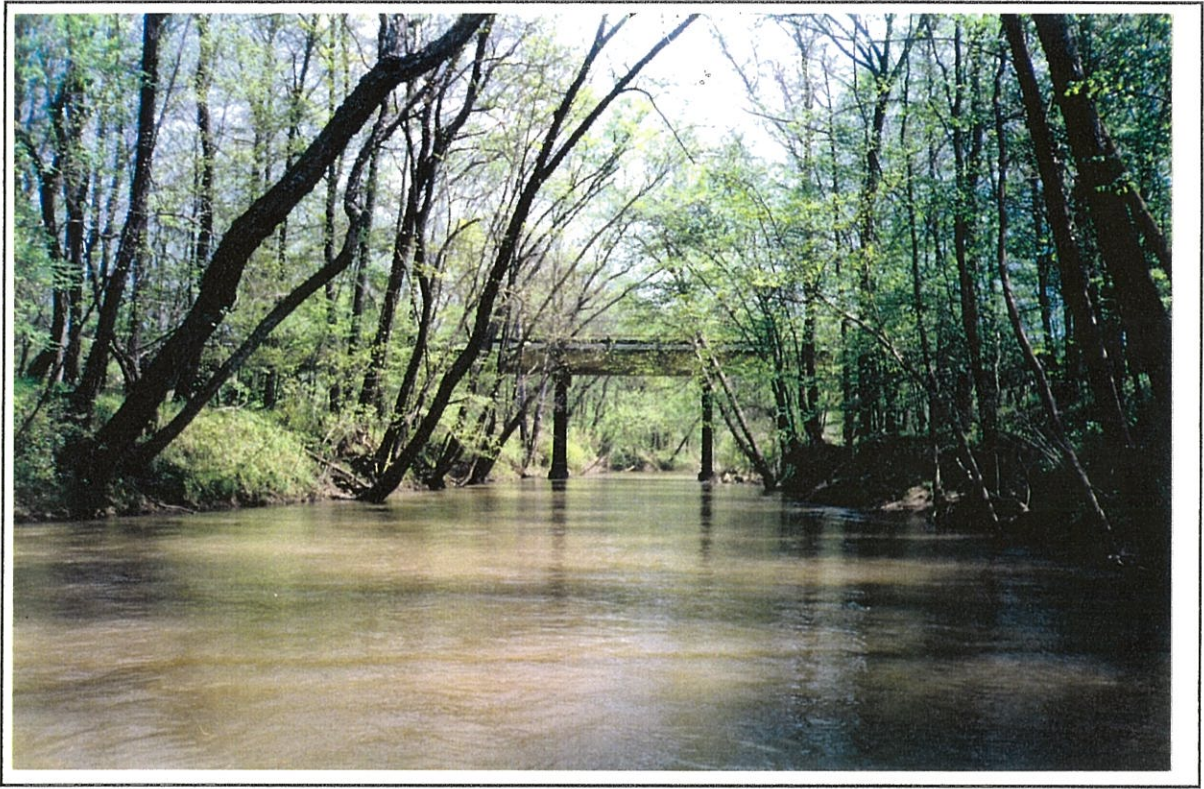
Figure 4. --Structure 124007200200 on Route SC 72, crossing the Sandy River in Chester County, South Carolina as viewed from 145 ft upstream (April 20, 1993).
