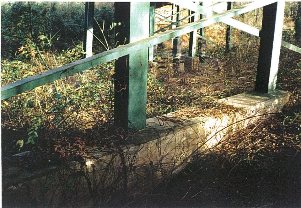
Photo 11: View eastward from west abutment.
