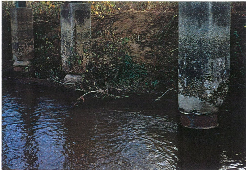
Photo 6: View of west bank - piles of bent 4.
