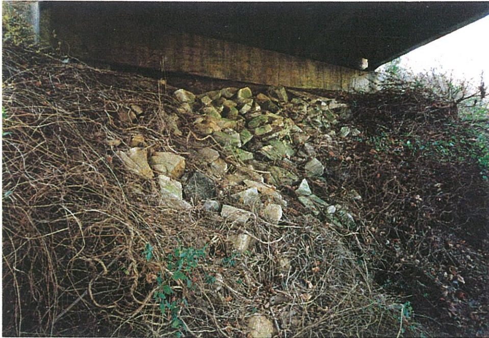
Photo 10: View of west abutment.
