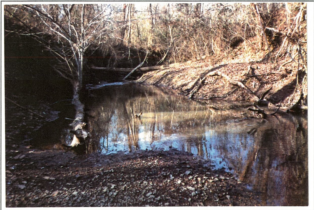
Figure 6. --Upstream channel as viewed from the approach cross section of structure 124007200700 on Route SC 72, crossing Rocky Creek in Chester County, South Carolina (February 11, 1992).
