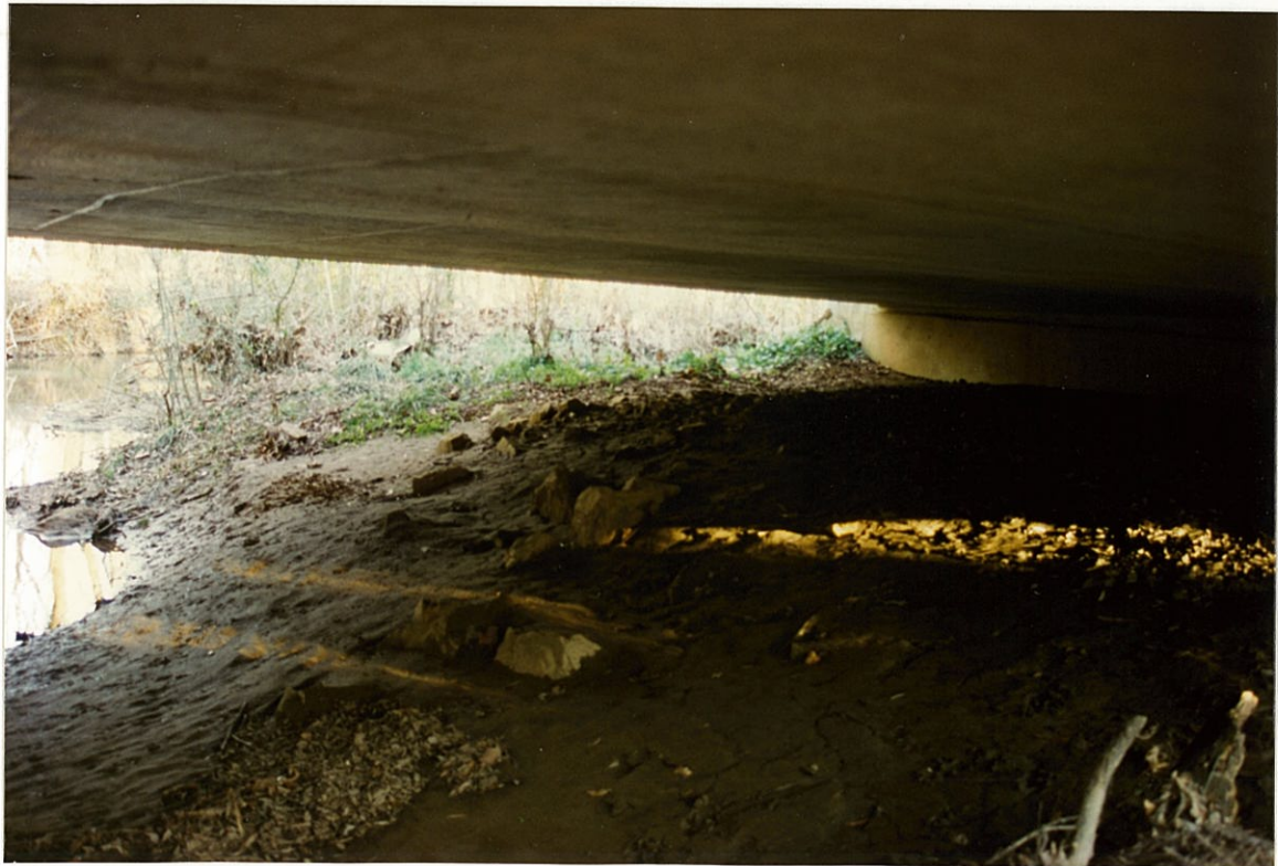
(10) LOOKING UPSTREAM AT SOUTHERN END BENT (#1).
