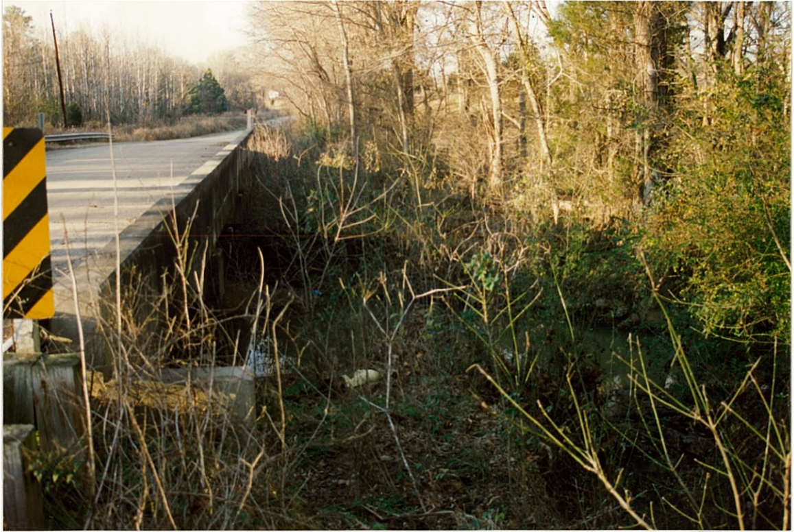
(5) UPSTREAM FACE LOOKING NORTH.
