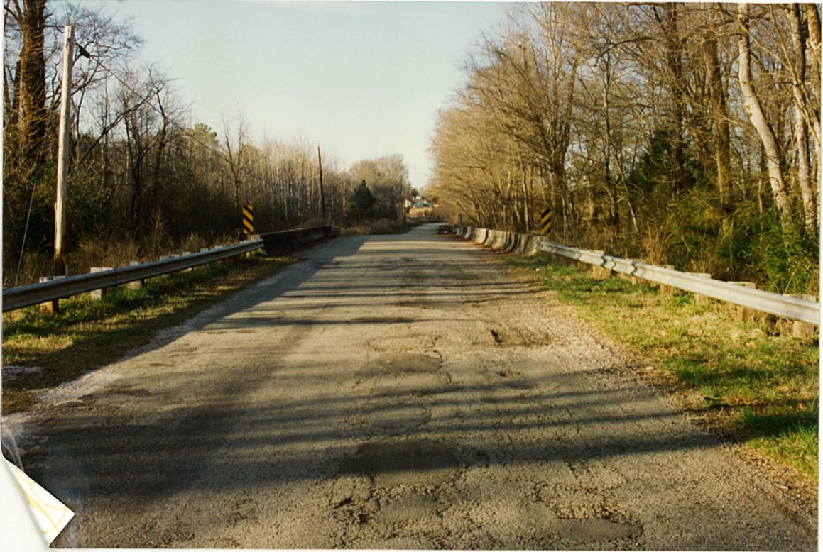
(1) LOOKING NORTH ALONG ALIGNMENT.
