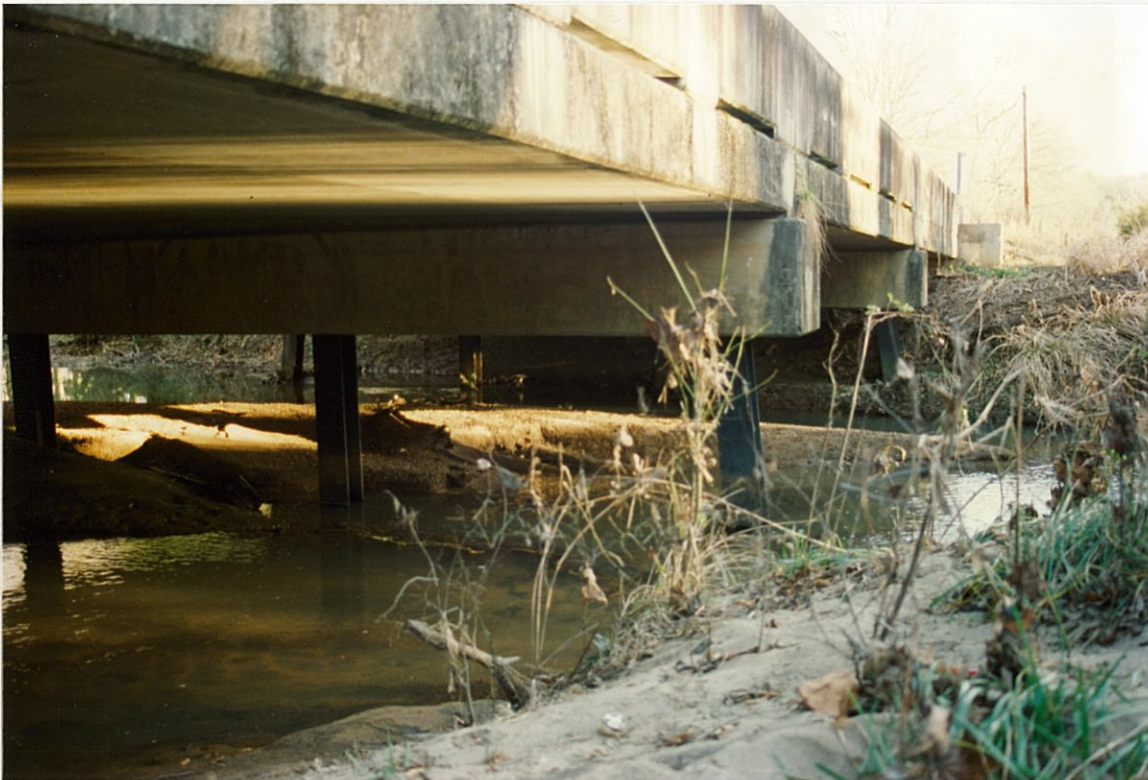
(8) LOOKING SOUTH ALONG DOWNSTREAM SIDE OF BRIDGE.
