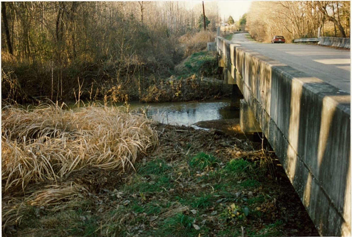
(6) DOWNSTREAM FACE LOOKING NORTH.
