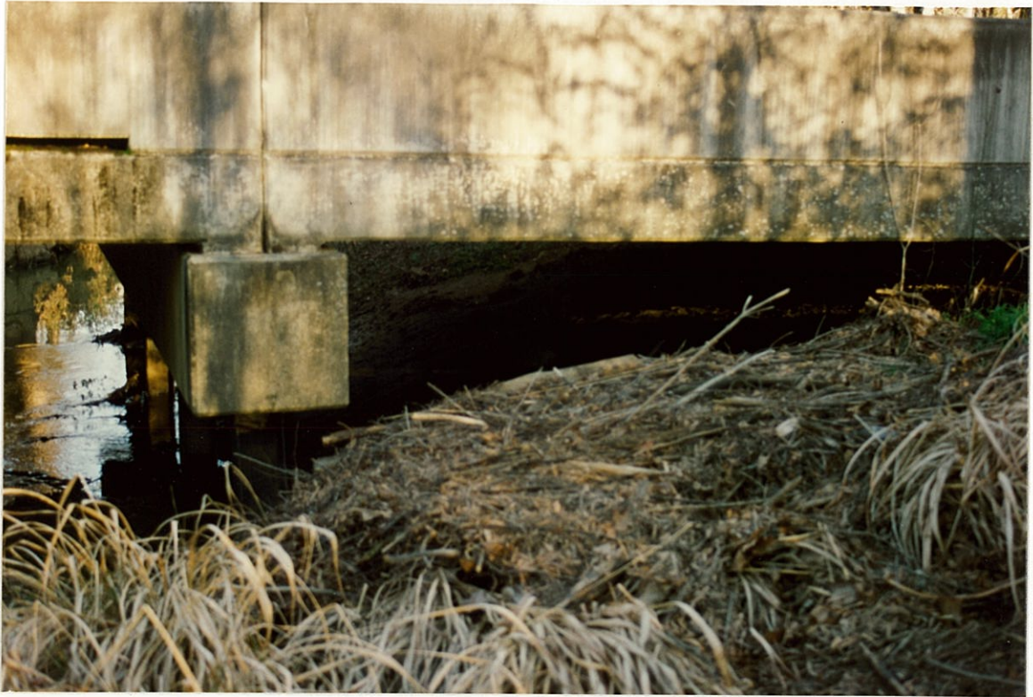
(9) LOOKING UPSTREAM AT BENT 2.
