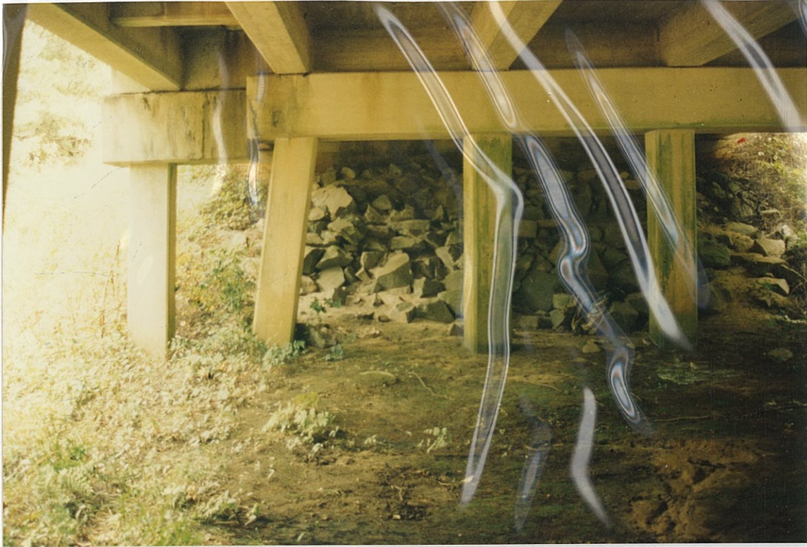
(7) Bent 1 and Bent 2
