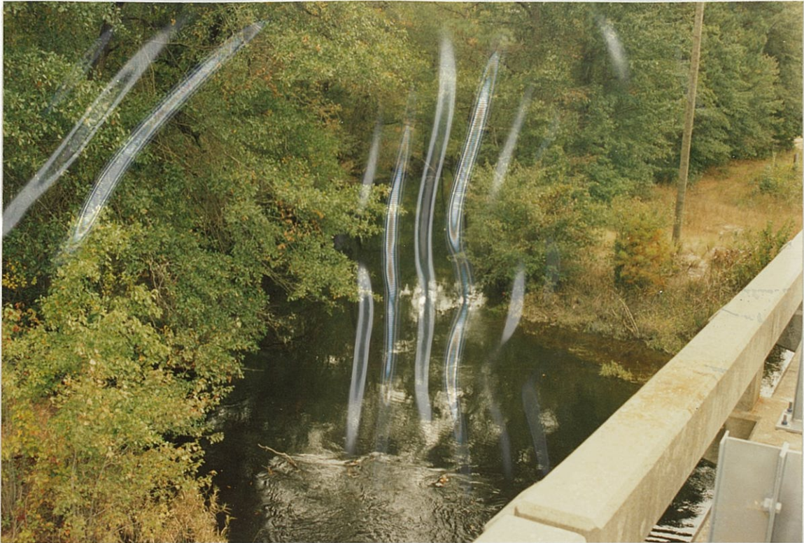
(5) Looking Upstream near Bent 6
