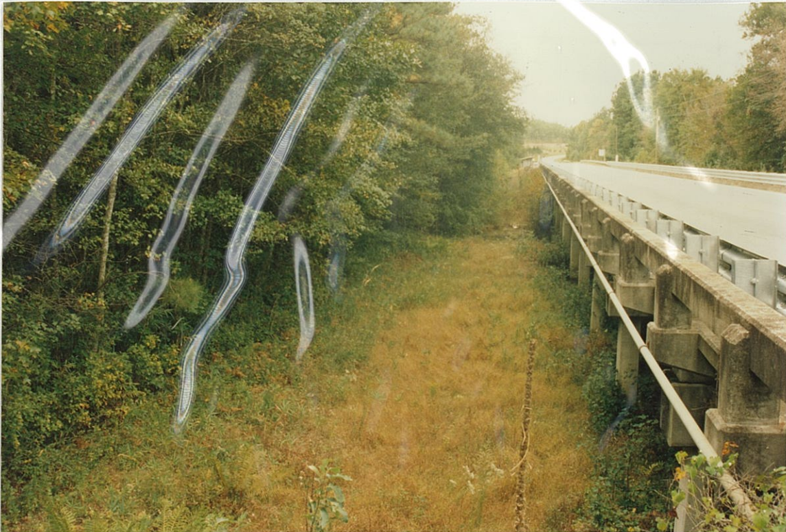
(9) Looking West along Downstream Face of Bridge
