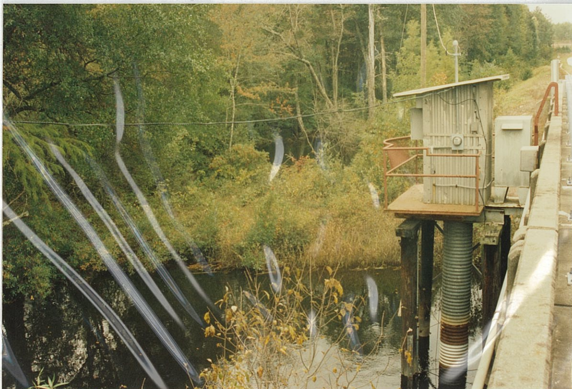
(10) Looking West along Downstream Face of Bridge at Main Channel
