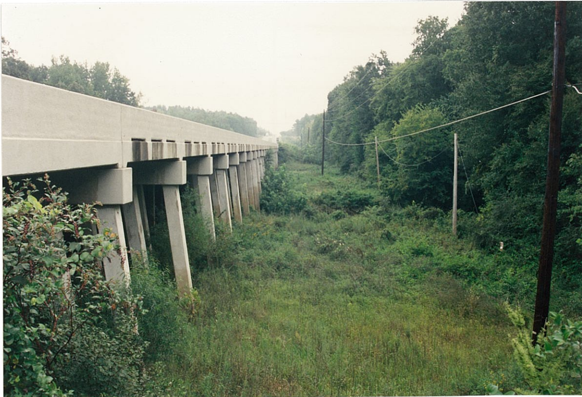
(12) Downstream side looking north
