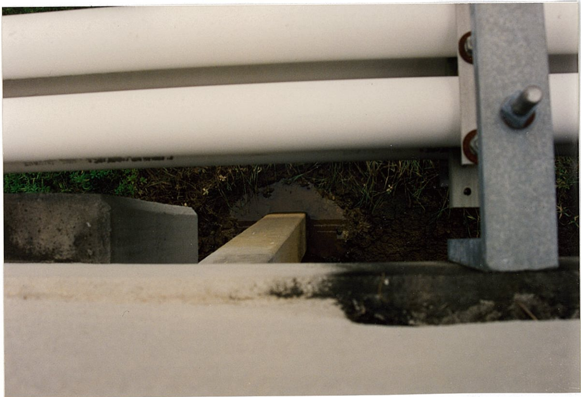
(8) Scour at Bent 23
