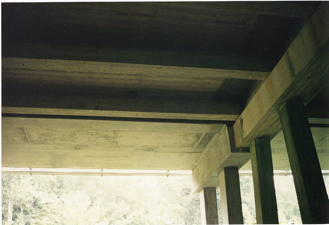
(6) Underside of original and widened bridge
