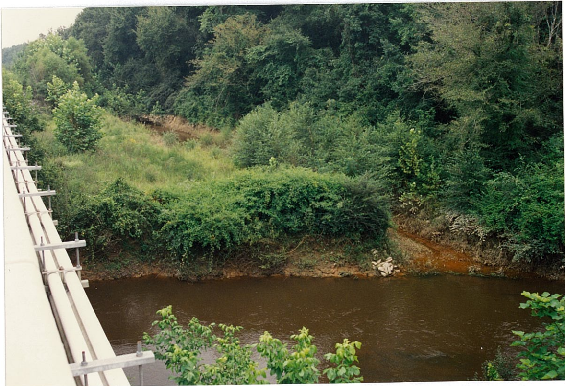
(4) Upstream side looking south
