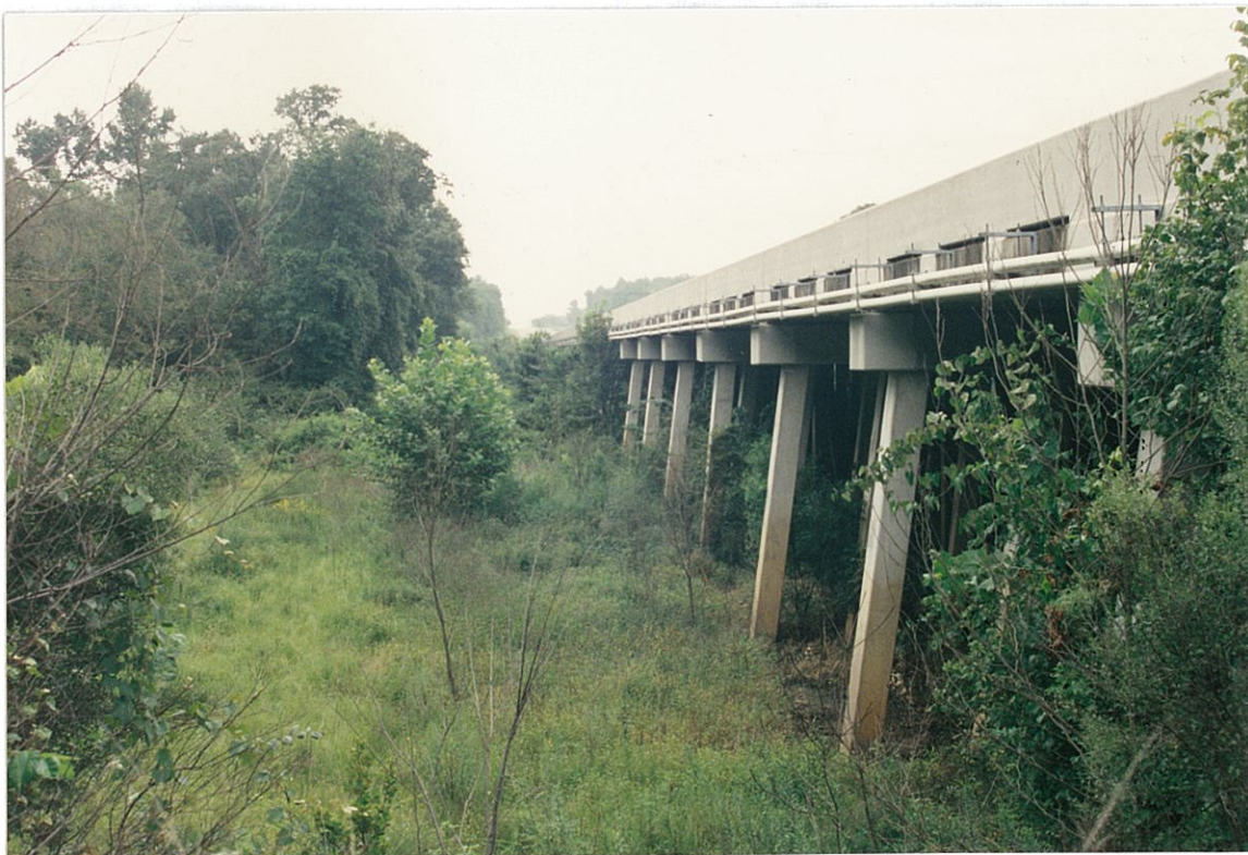
(2) Upstream side looking north
