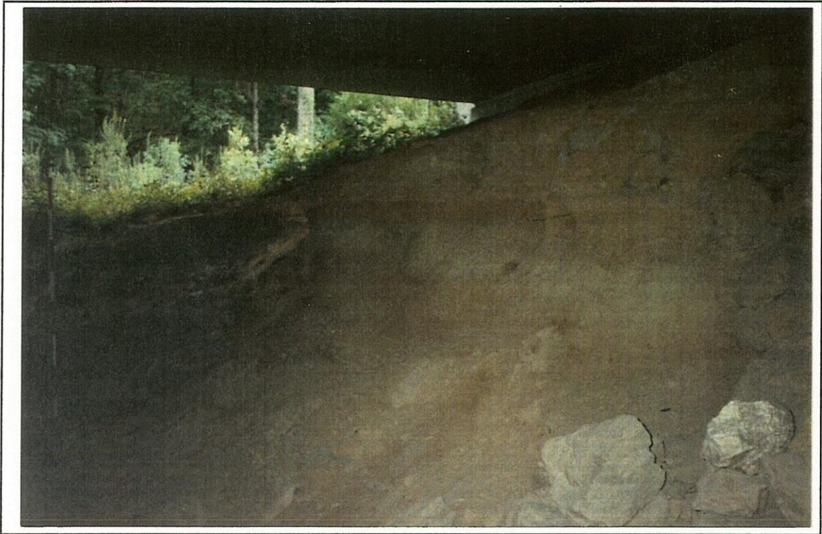
**Figure 8.**--Severe erosion of the right abutment of structure 134000900400 on Route SC 9, crossing Thompson Creek in Chesterfield County, South Carolina (September 4, 1990).
