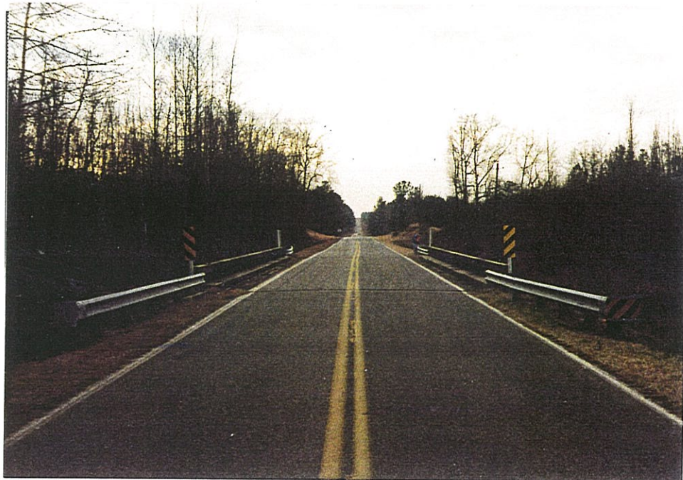
Photo 2- View looking south on Route SC-102.
