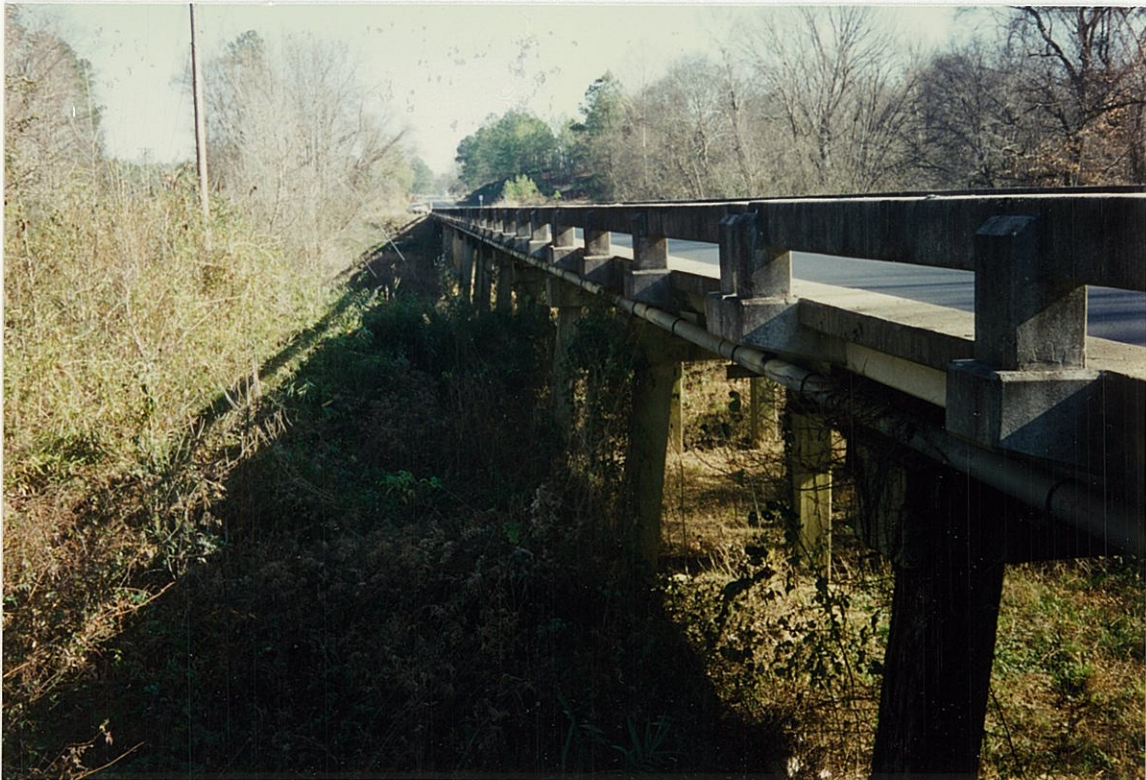
(8) Upstream Face Looking East
