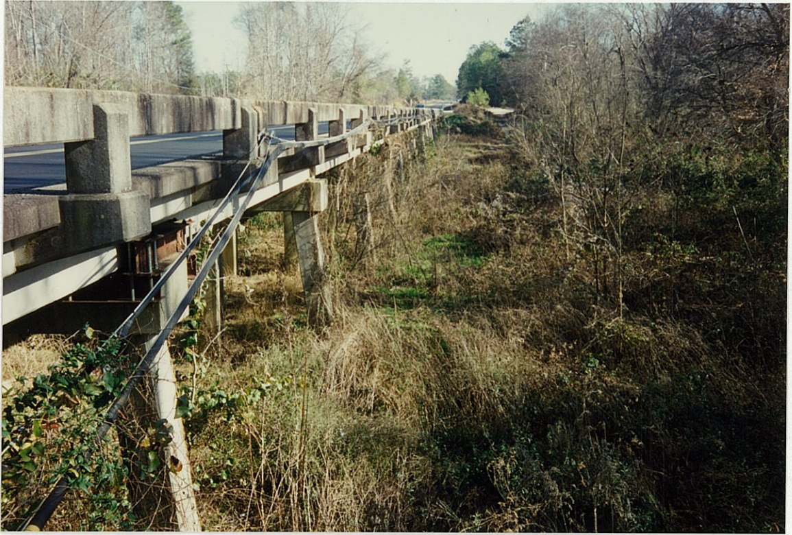
(9) Downstream Looking East
