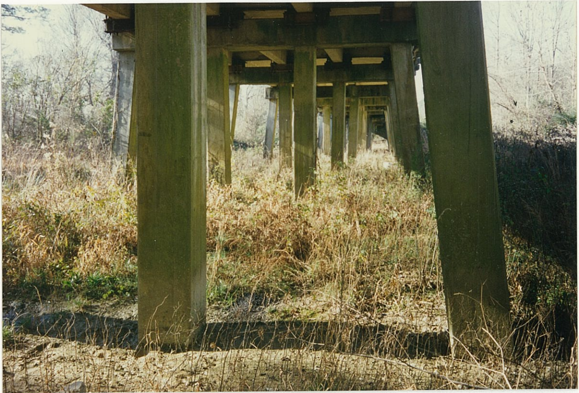
(5) Looking West Under Bridge
