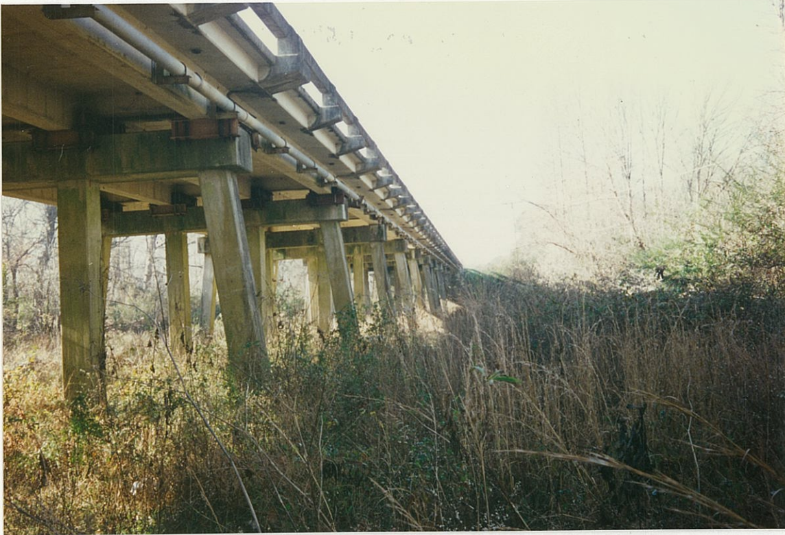
(3) Looking West Across Upstream Face
