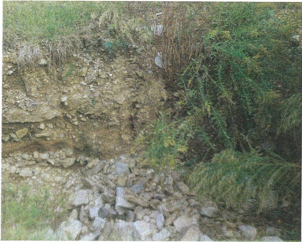
**Photo 11:**      *Erosion from surface runoff on upstream side of north abutment.*
