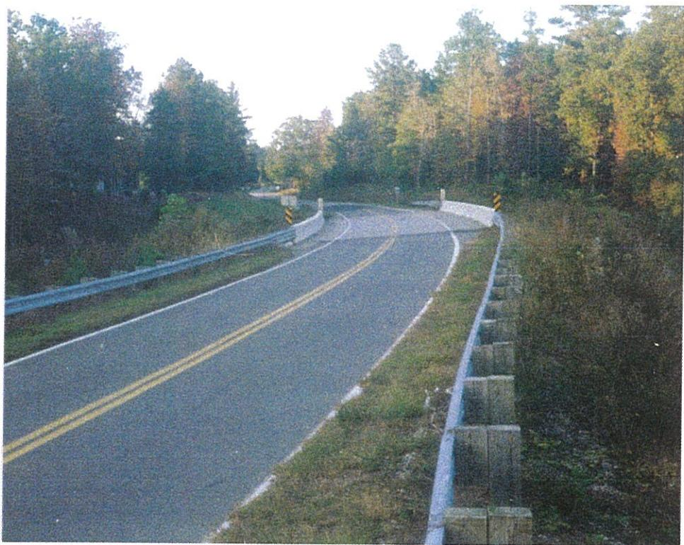
*Photo 1:* View looking north. Note superelevation.
