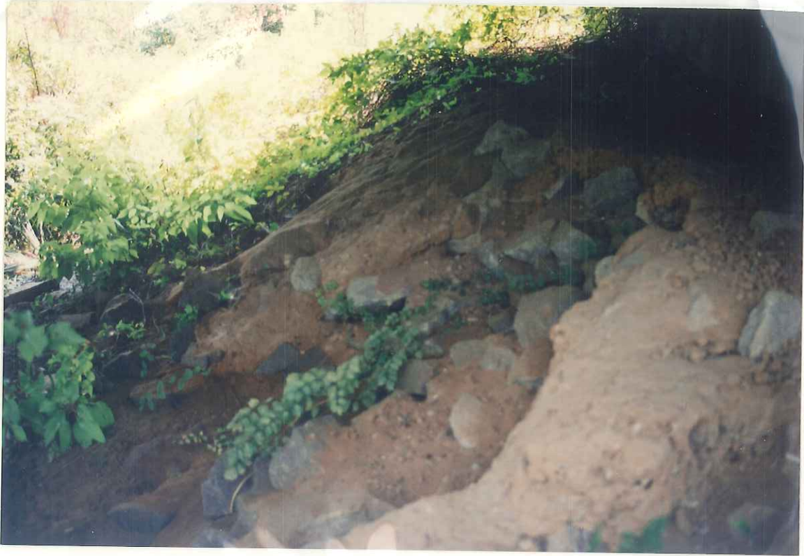
(11) Looking downstream at End Bent 2
