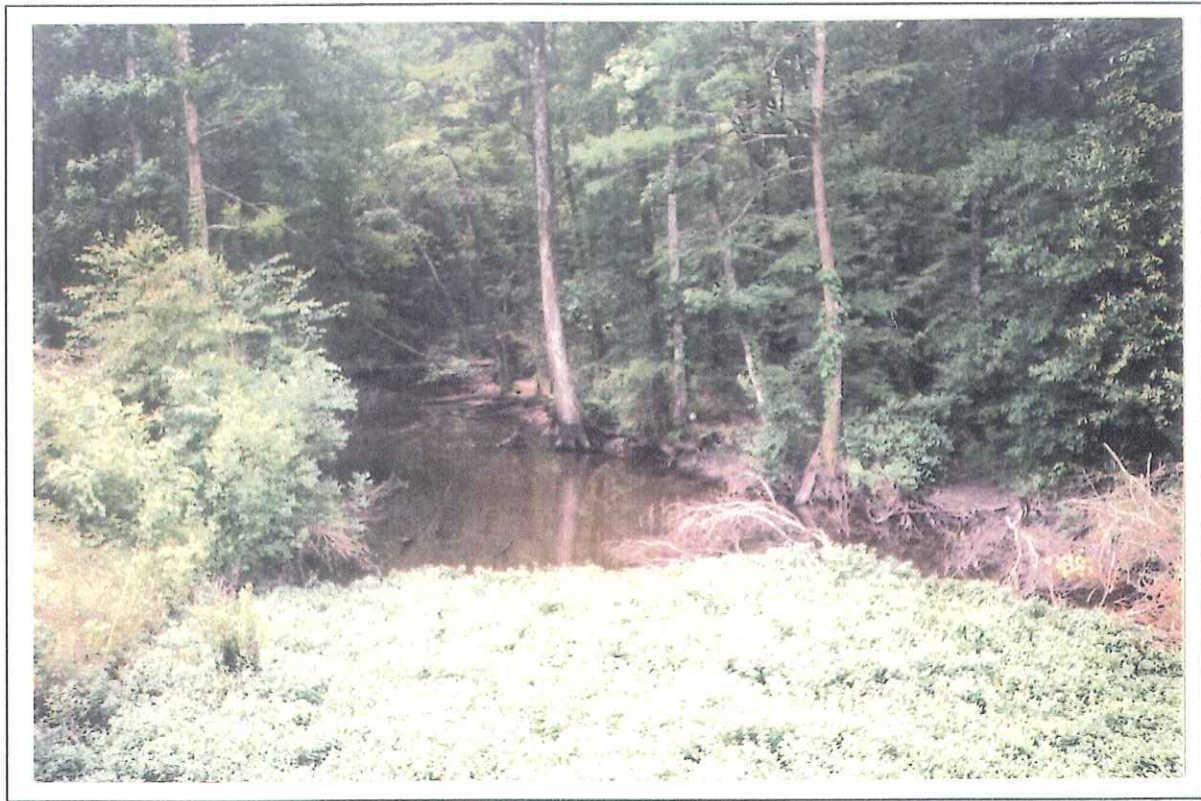
Figure 7. --Downstream channel as viewed from structure 182007800100 on Route US 78, crossing Cattle Creek in Dorchester County, South Carolina (May 24, 1990).
