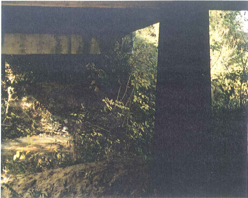
Photo 8: View looking at west bank/abutment from east bank of main channel.
