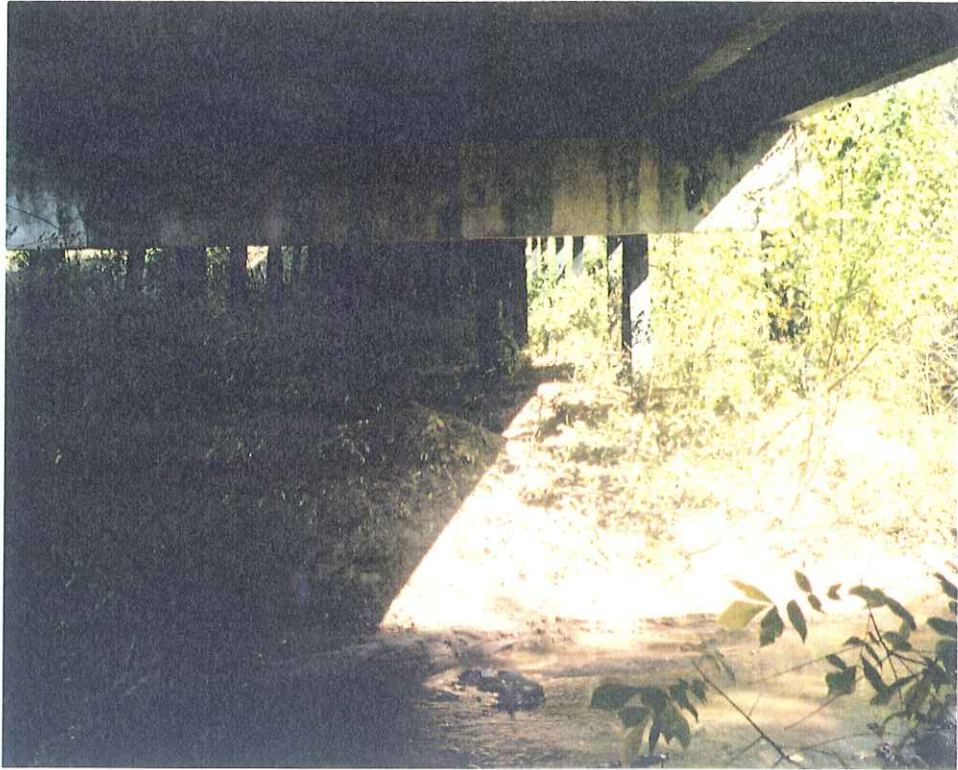
Photo 7: View looking at east bank of main channel from west bank/abutment.
