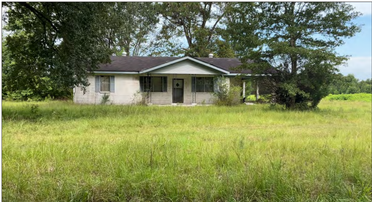
Figure 5.46 View of SHPO Site No. 1387 facing east.
