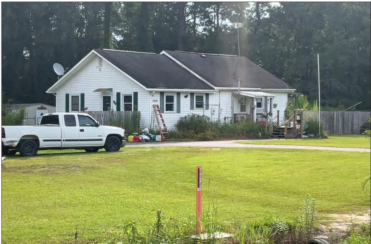
Figure 5.56 View of SHPO Site No. 1397 facing east.
