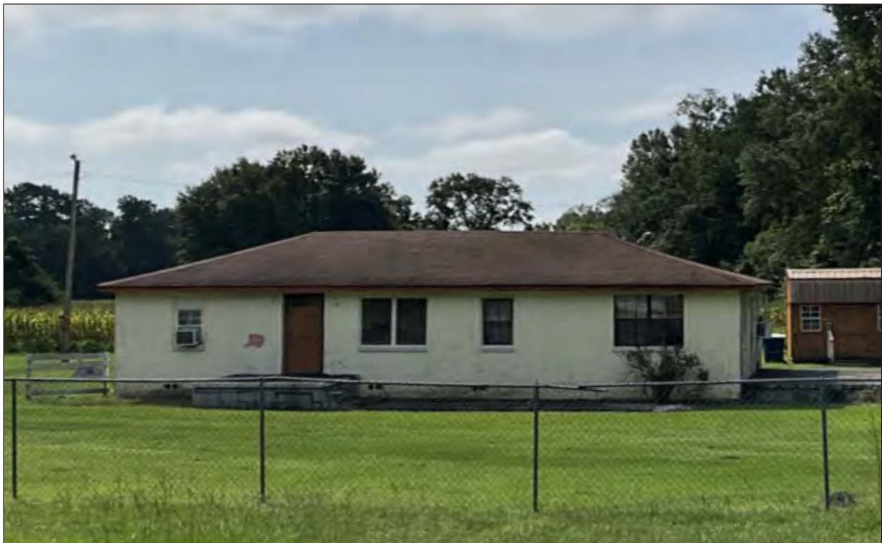
Figure 5.68 View of SHPO Site No. 1410 facing southeast.
