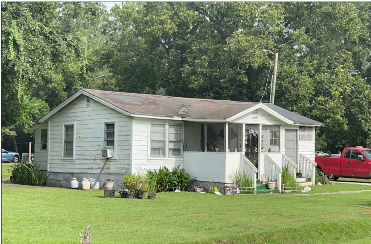
Figure 5.70 View of SHPO Site No. 1507 facing east.
