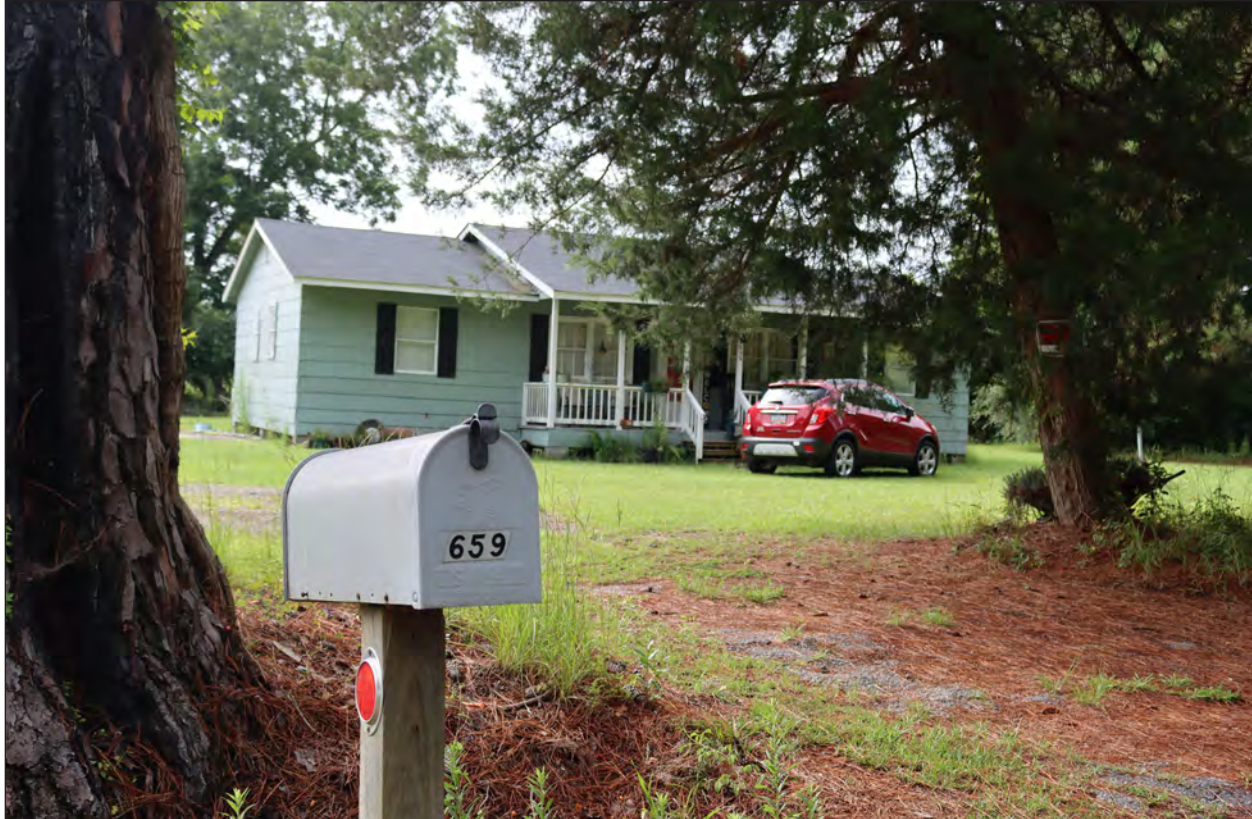
Figure 5.5 View of SHPO Site No. 1339 facing east.
