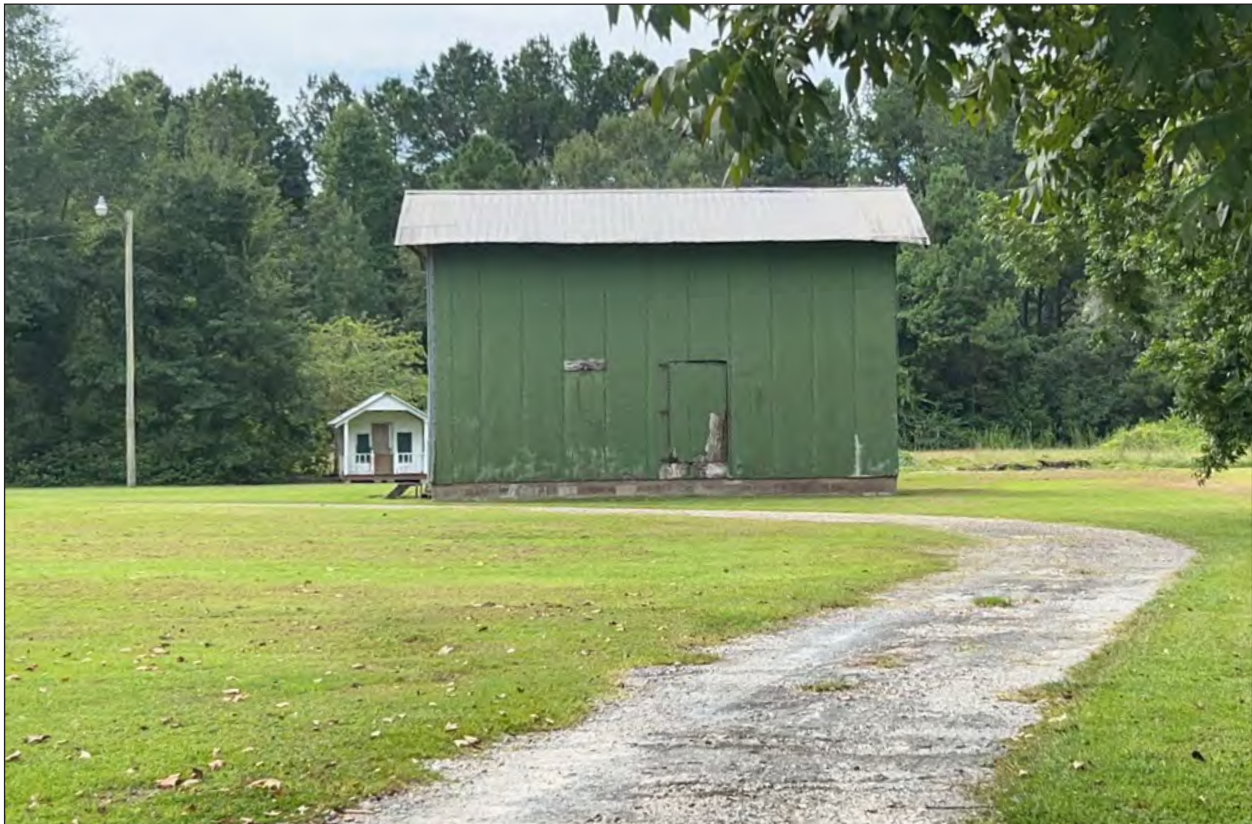
Figure 5.66 View of SHPO Site No. 1408 facing east.
