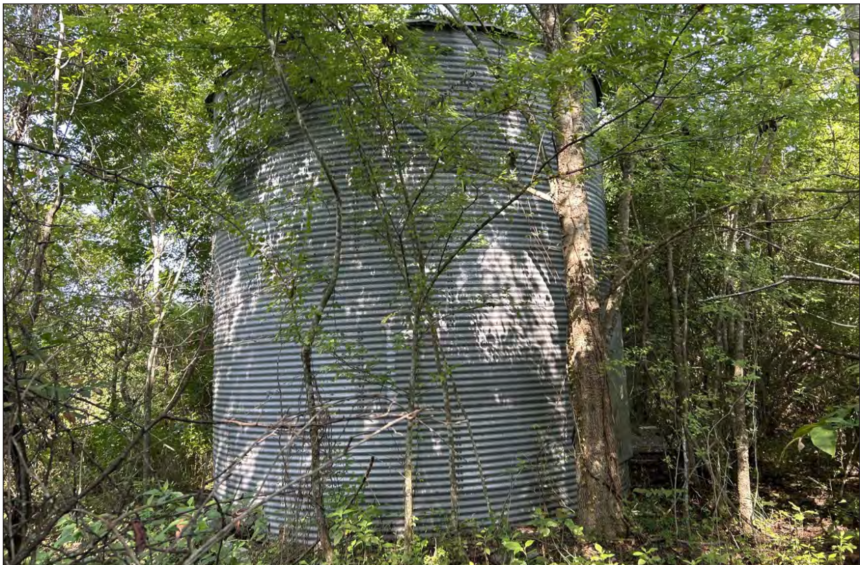
Figure 5.44 View of SHPO Site No. 1385 facing east.
