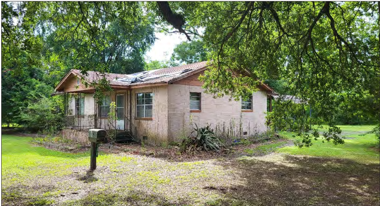
Figure 5.47 View of SHPO Site No. 1388 facing east.
