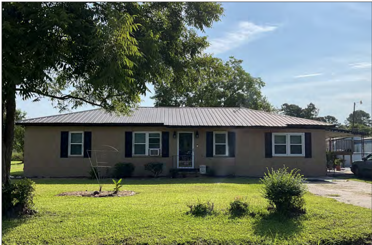
Figure 5.57 View of SHPO Site No. 1399 facing east.
