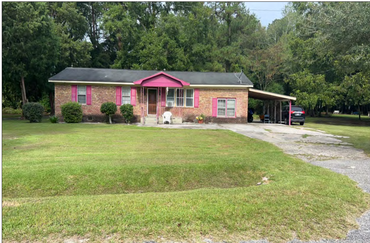
Figure 5.76 View of SHPO Site No. 1512 facing east.
