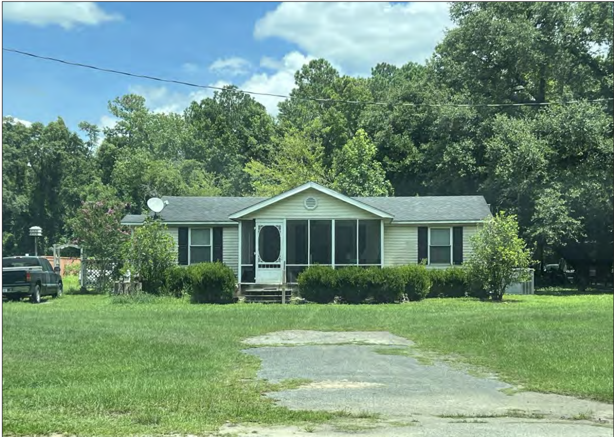
Figure 5.60 View of SHPO Site No. 1402 facing east.
