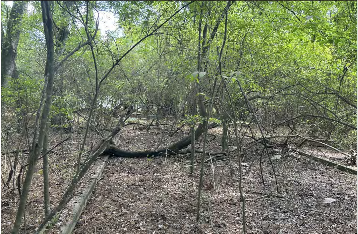
Figure 5.29 State of concrete foundations at 38DR543 in July 2024 facing east.
