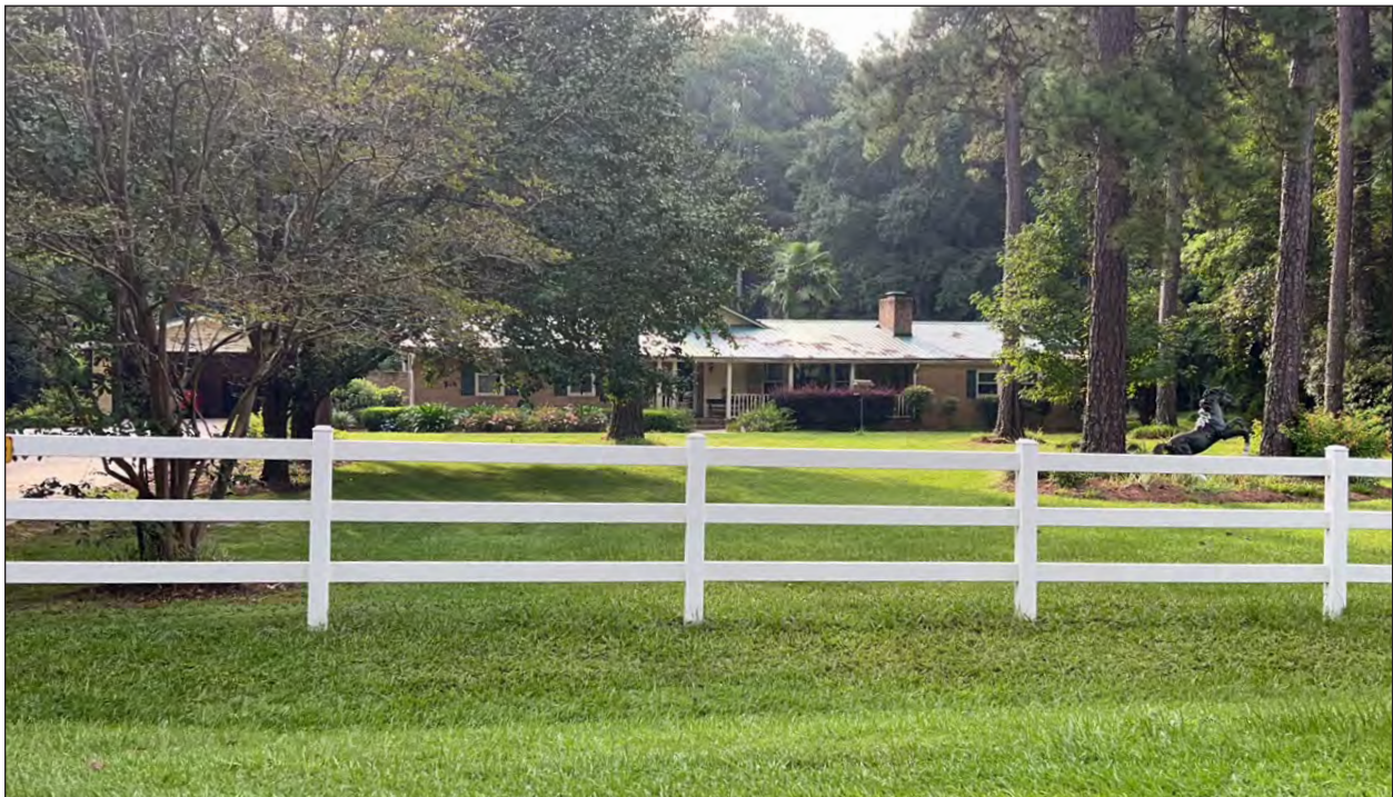
Figure 5.45 View of SHPO Site No. 1386 facing east.
