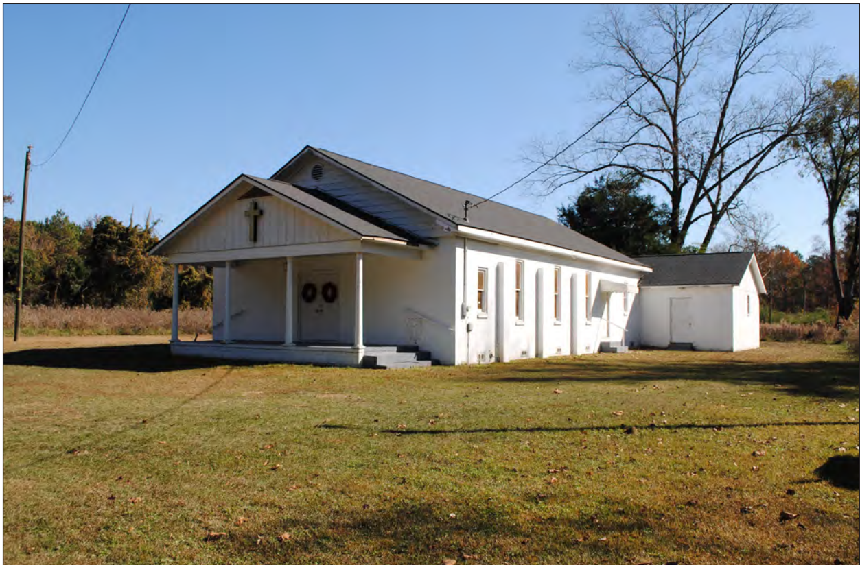
Figure 5.73 View of SHPO Site No. 1510 facing east.
